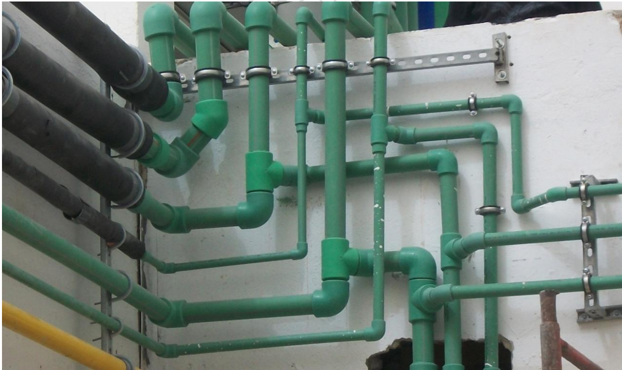
PPR Piping for Supply Water
