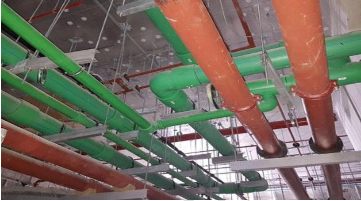
PPR Piping for Supply Water
