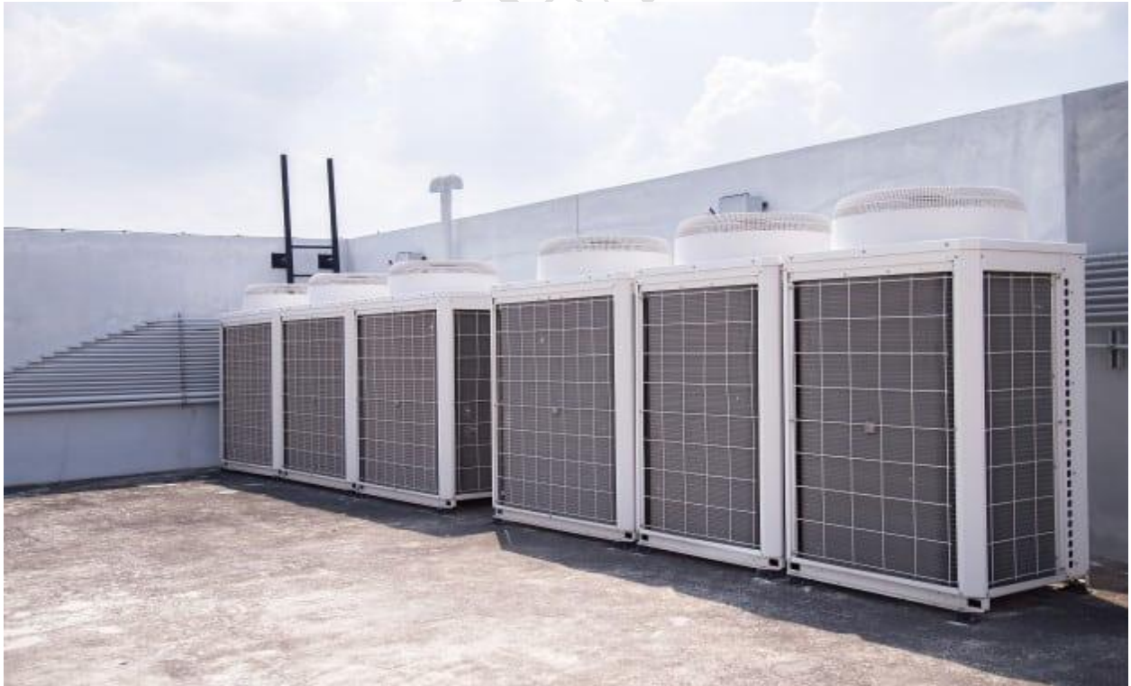
VRV Unit Installation
