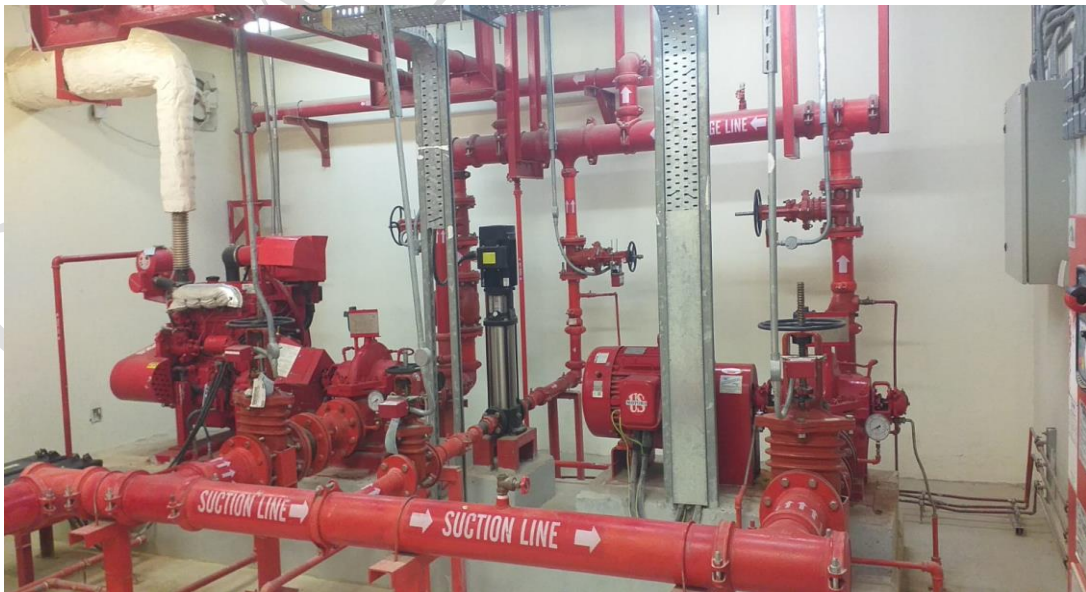
Fire Fighting Work
